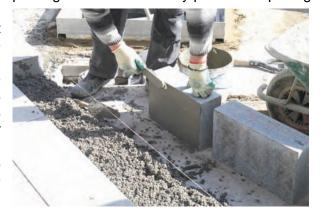
Paving units are to be beaten with the maul firmly to line and level without delay and thereafter they are not to be disturbed. The short level is frequently used to slide across the freshly laid paving units, the check for lips. The long level should be frequently used to check level over wider areas.
