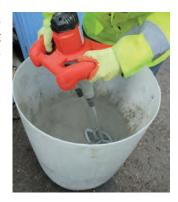
Mixing should be made using a powered paddle mixer, either hand-held or stationary. Manual mixing is not good practice due to the risk of incomplete blending.
